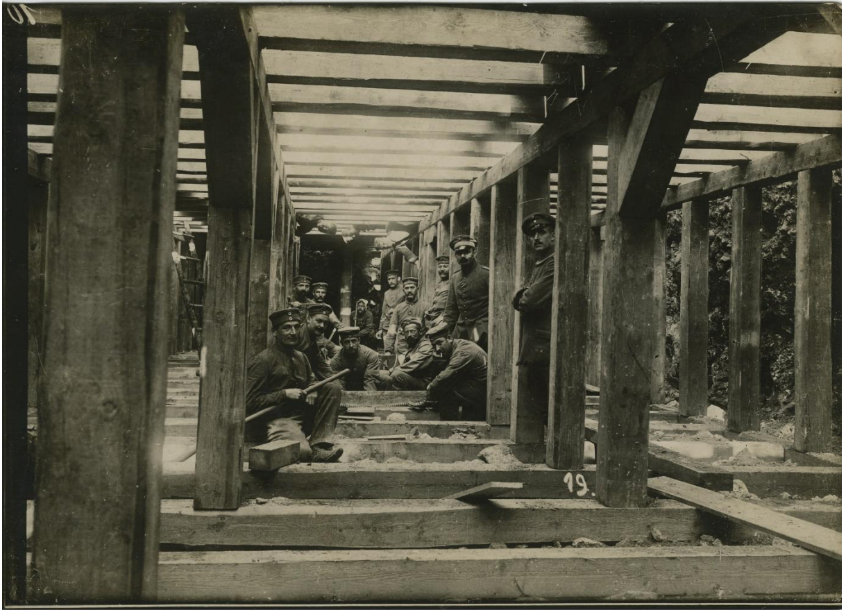
A large dugout under construction
